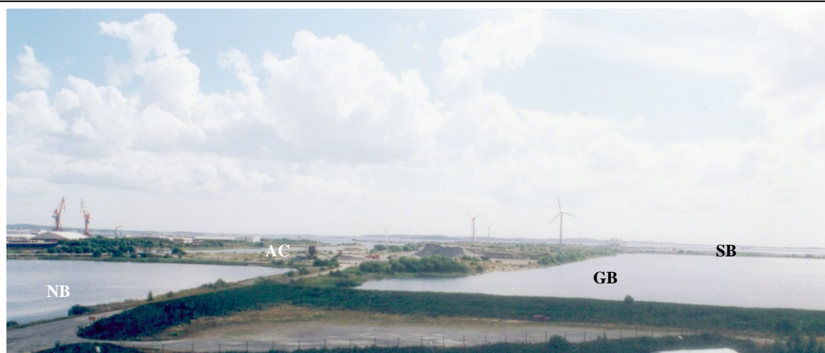
A view towards the south of the Bay of Torslandaviken. Brackish water is entering from the Rivö Fjord in the back ground through the Arendal Channel (AC) into the Northern Basin (NB) and then into the Great Basin (GB) . The embankments of the Southern Basin (SB) are bordering towards the south. (Photo 2000-07-25).
